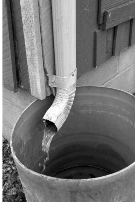
Suggested rain barrel design.
