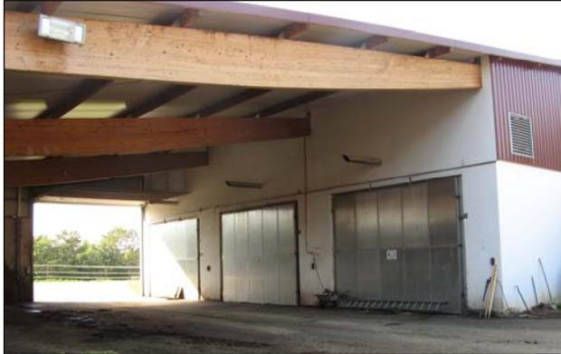
The percolate tank is to the left of the building. PV panels located on the large roof provide an additional source of renewable energy. Access doors to the three vessels face a covered mixing area. Newer units have replaced the single hinged access doors with smaller double doors that open in both directions.
