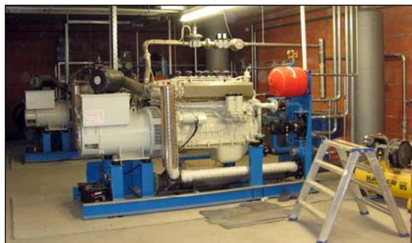
Two 178 kW CHP units are located over the back of the first vessel. The system was producing at 360 kW during our visits but earlier in the year production was as low as 190 kW due to problems with the biology of the system.
